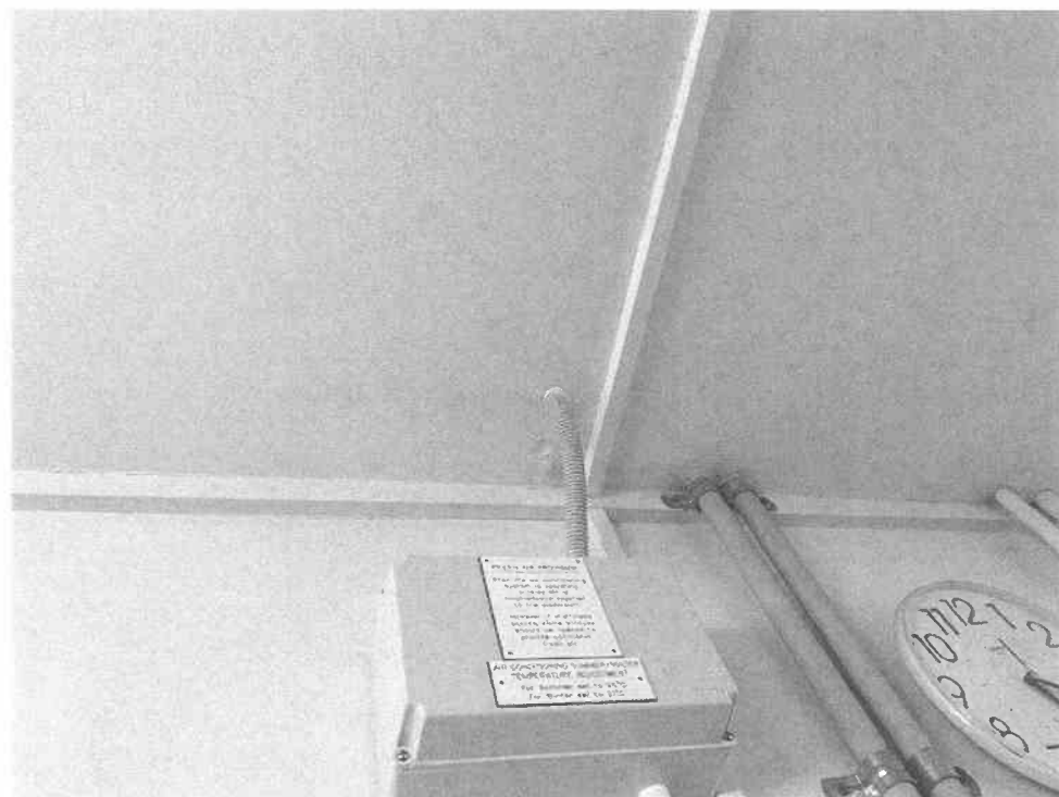
Site Image 7: Edges of penetrations sealed with silicone.
