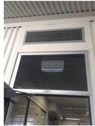
Figure 5 – C Block Typical Fresh Air Louvre
