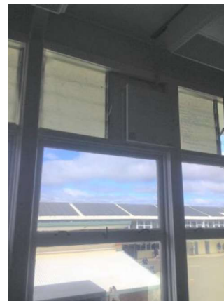
Figure 5 – C Block Faulty Wall mounted Filter / Fan Unit
