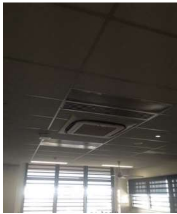
Figure 4 – C Block AC Cassette with Fresh Air Grilles
