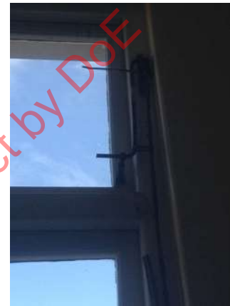
Figure 3 – A Block Zip Tied Opening Mechanism
