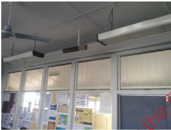
Figure 1 – A Block Under Ceiling Heater Bar
