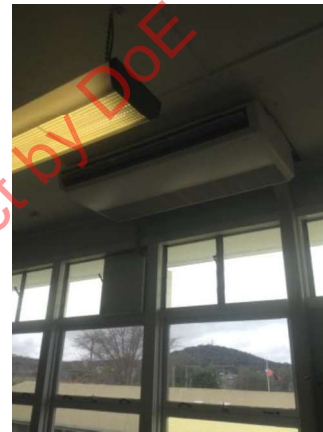
Figure 2 – A Block Under Ceiling AC Unit
