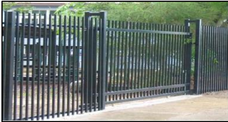
Picture 6.1: Type 1 Security Fencing Sliding Gate
