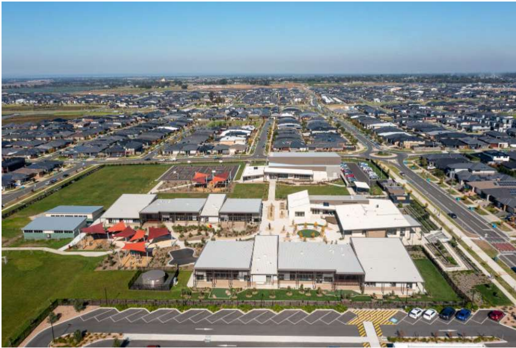
Ramlegh Park Primary School, Clyde North – opened 2021
